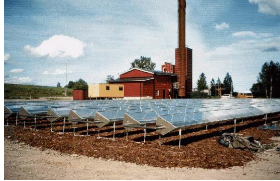
Figure 1.15: Construction principle of the MaReCo (Maximum Reflector Collector) with stand-alone MaReCo field of A_{ap} = 500 \text{ m}^2 and row length of 40 m constructed in 1999 supporting a bio fuel burner in Torsåker, Sweden. Left picture from (Adsten et al. 2004, p. 201), right picture from (Adsten 2002, p. 41).
