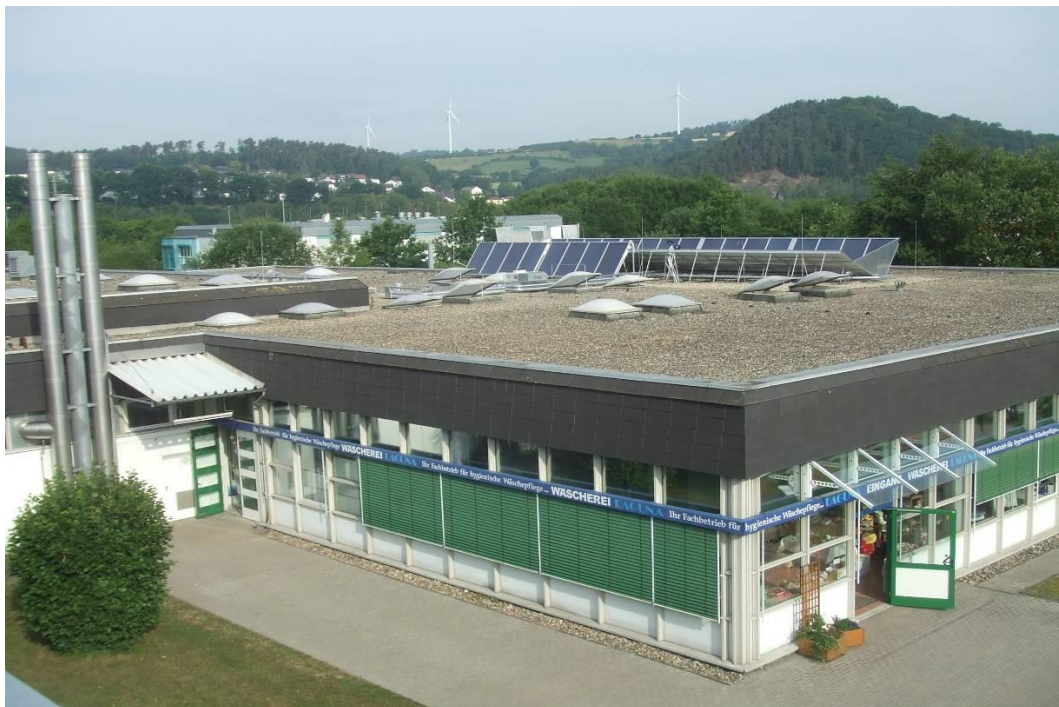
Figure 5.1: Laundry Laguna with production and service building (front), boiler house (left) and solar thermal installation. Picture: Wagner & Co. Solartechnik
