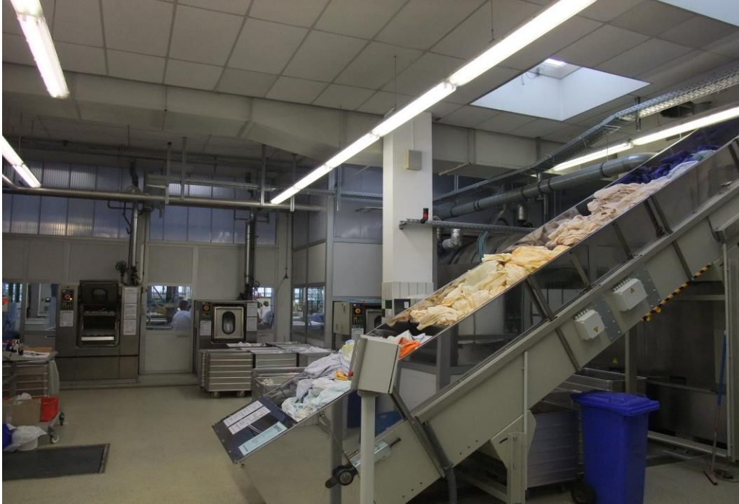
Figure 5.2: Unclean side with three industrial washing machines (left: 50 kg charging weight; central background: two machines à 25 kg) and the batch tunnel washer (right background) with its charging conveyor belt (front). All these devices are heated by steam injection. Their outlet is on the clean side, where the laundry is dried and finished.
