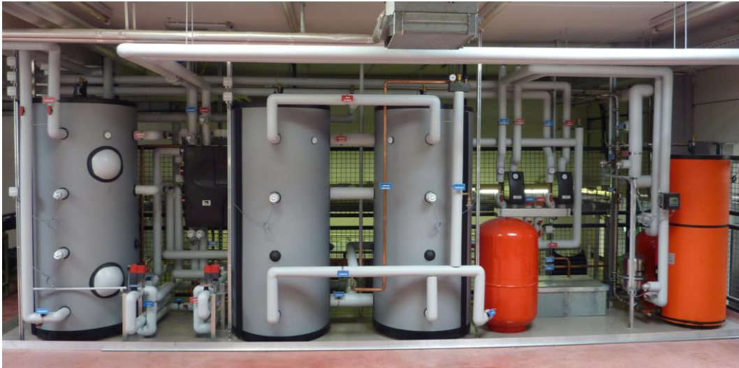
Figure 5.7: Centralized components of the RefleC pilot system with monitoring sensors.
