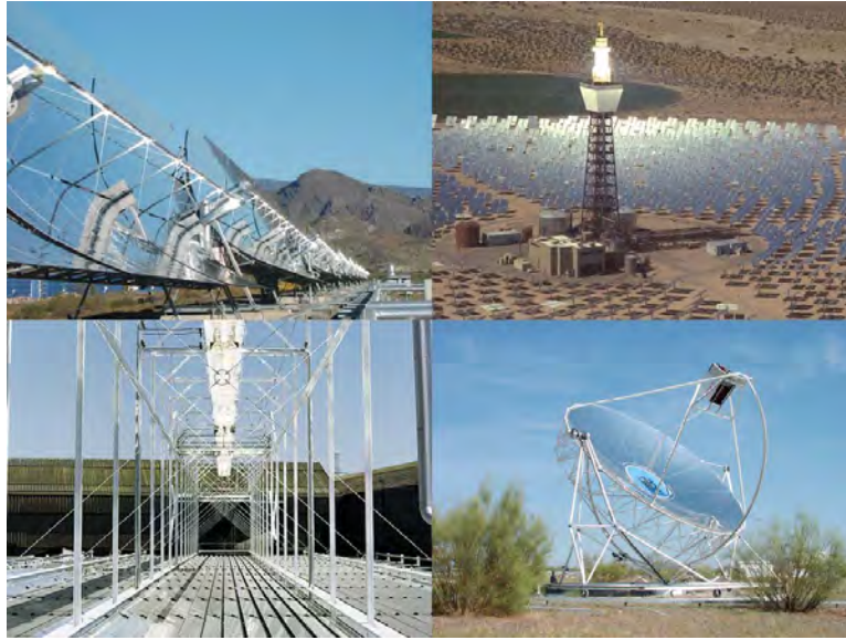
Fig. 2.2: Parabolic Trough (upper left), Linear Fresnel (bottom left), Solar tower (upper right) and Solar Dish (bottom right) [17]
