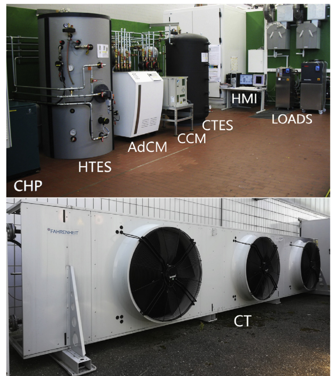
Figure 1. (above) Microscale trigeneration plant at INES with Compression Chilling Machine (CCM) (below) Cooling tower (CT).
