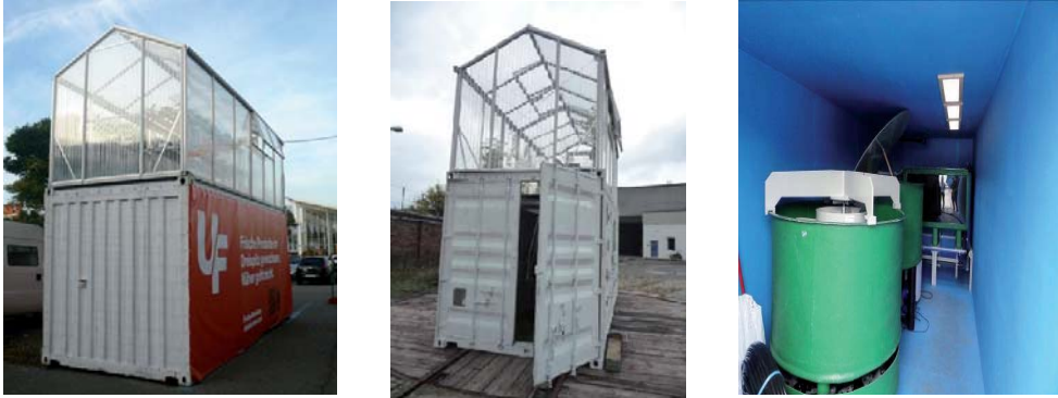
Figure 53: Container Farm aquaponics – mobile urban showcases with fish tank at ground level and greenhouse above. Left: Urban Farmers, Basel. Middle and Right: Rebuild model by ECF, Berlin
