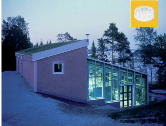
Figure 57: Stensund Wastewater Aquaculture – Trosa community, Sweden
